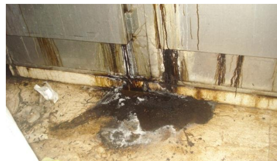
Figure: 6- purified fluids damaging refrigerators
